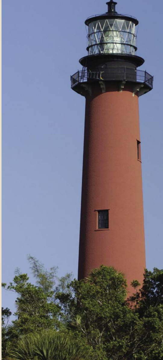
The Jupiter Lighthouse is known for its distinctive red color, which was painted on after its bricks began to fade.
